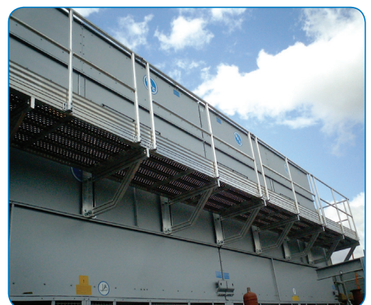
BAC model VXI closed circuit cooling tower with discharge sound attenuation package
