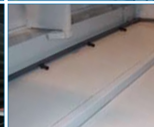
Sloped basin with sump sweeper piping*
