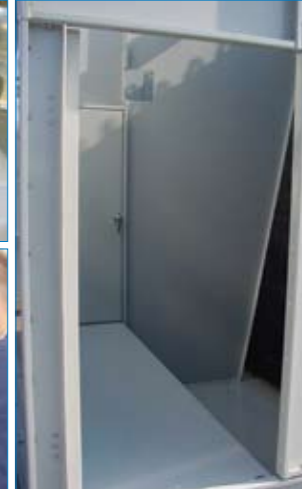
Inward swinging access door and internal walkway*
