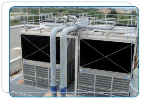
Combined Inlet Shields retrofitted to the top half of BAC S3000 cooling towers with old style louvres at the bottom
