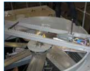
Mechanical equipment removal*
