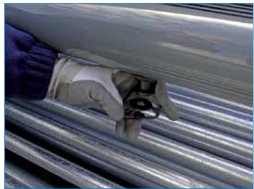
Inspecting Spray Distribution Nozzles
