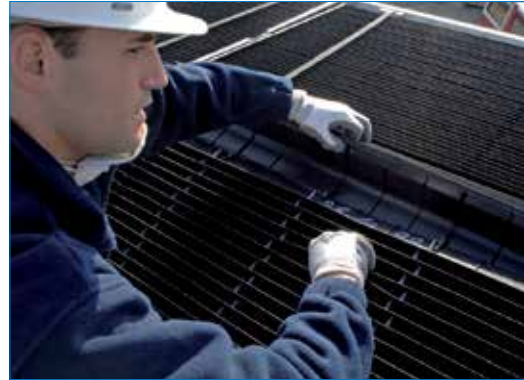
Inspecting Drift Eliminator
