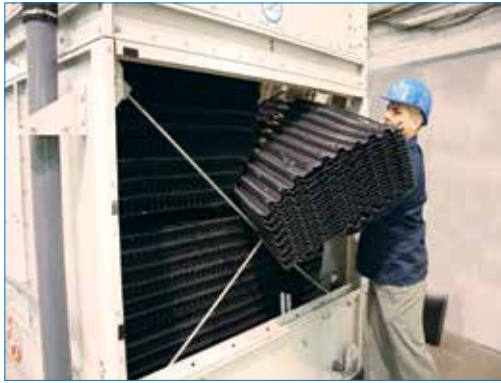
Installing Retrofit Kit
