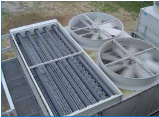
Pressurized Spray Water Distribution
