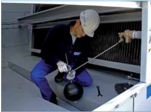
Mechanical Water Level Control
