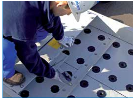
Hot Water Basin with Gravity Water Distribution
