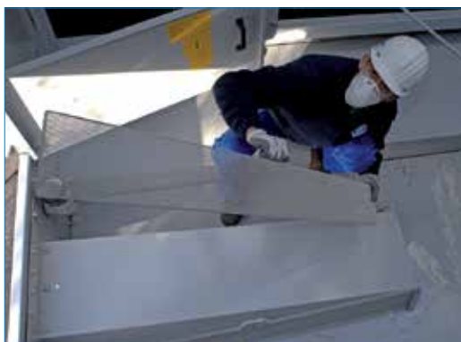
Inspecting Cold Water Basin Strainer
