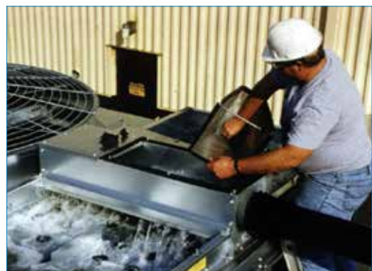
Hot Water Basin Strainer Cleaning
