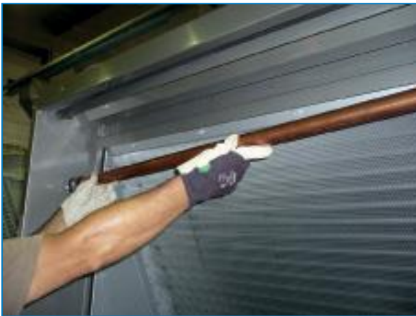
Remove Copper Waterfeed Pipe
