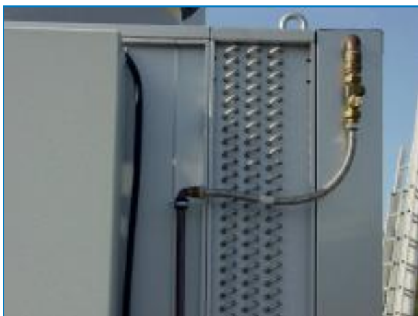
Waterfeed Assembly connected to City Water Connection with Flexible Pipe
