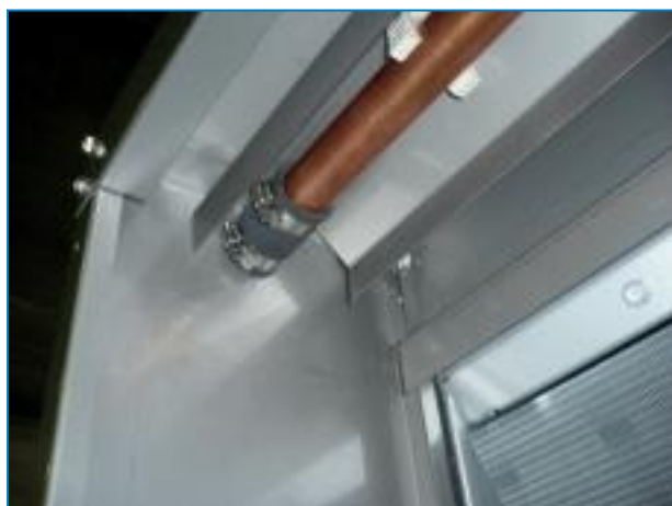
Flexible Sleeve Connection
