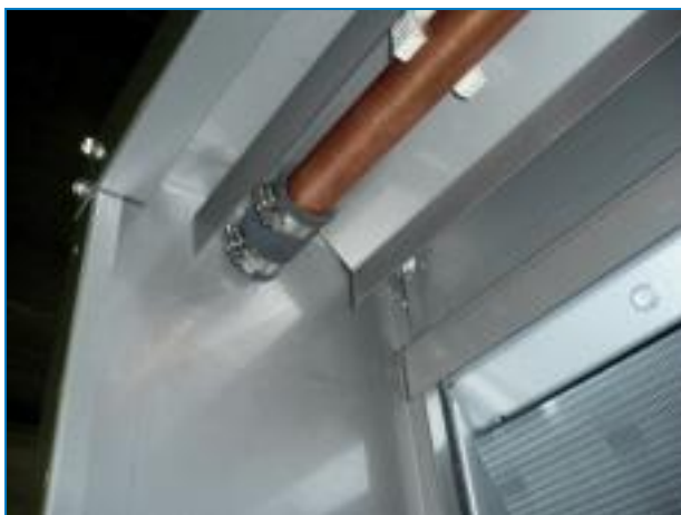
Flexible Sleeve Connection with Sleeve Clamps
