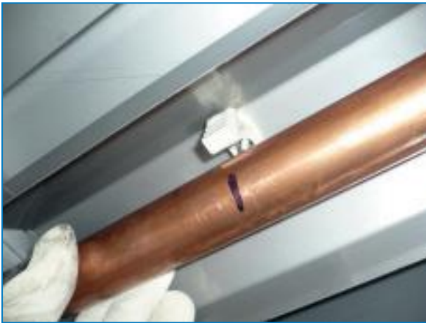
Alignment of Waterfeed Pipe
