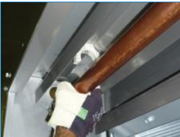
Release Copper Collector from Plastic Holders
