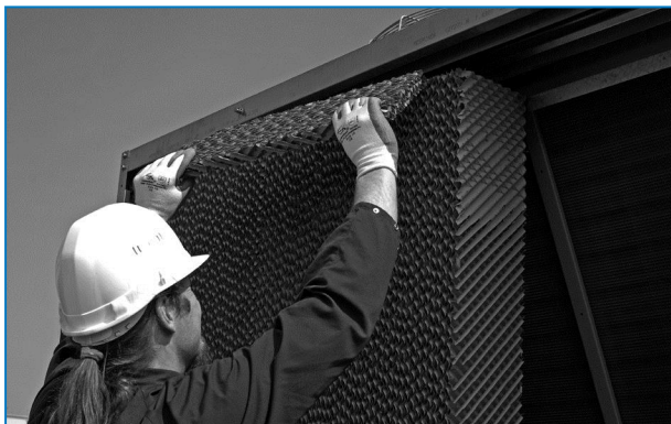
Removal Water Distribution Pads
