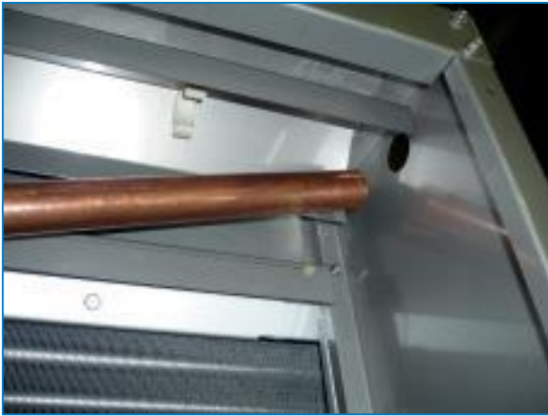
Installation of Copper Waterfeed Pipe
