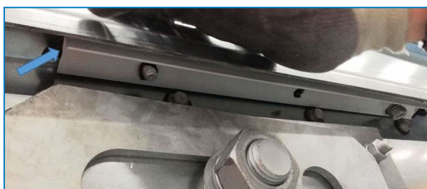
Installed Sealing Profile
