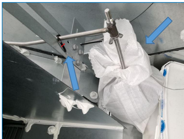
Fixation and wrapping of Float ball
