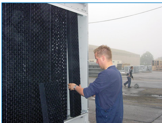
Remove Combined Inlet Shields
