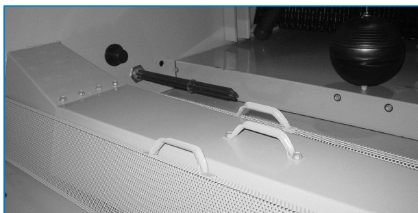
Cold Water Basin and Basin Strainer
