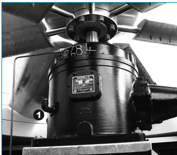
Single Reduction Gear Drive
