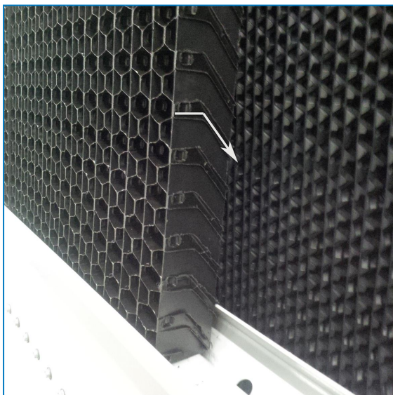
Orientation of the combined inlet shield
