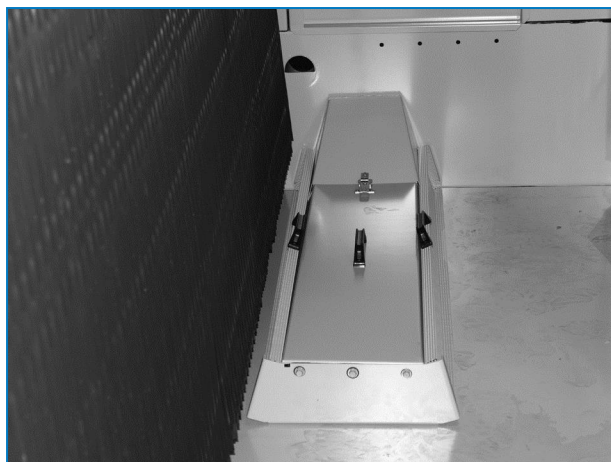
Cold Water Basin and Basin Strainer
