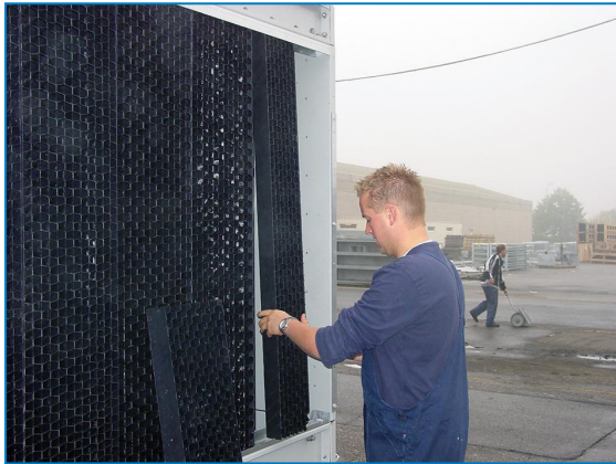
Remove Combined Inlet Shields
