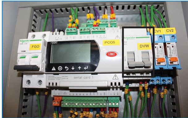
Pad Maintenance Switch (DVW) for EC fans
