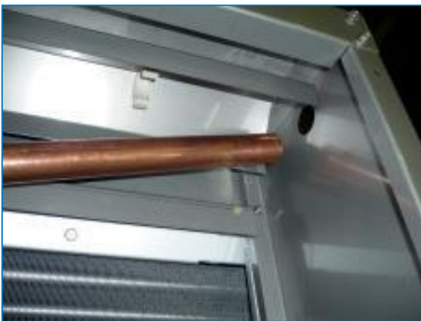
Installation of Copper Waterfeed Pipe
