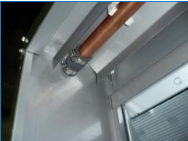
Flexible Sleeve Connection with Sleeve Clamps
