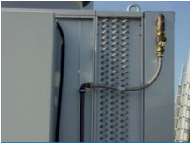
Waterfeed Assembly connected to City Water Connection with Flexible Pipe
