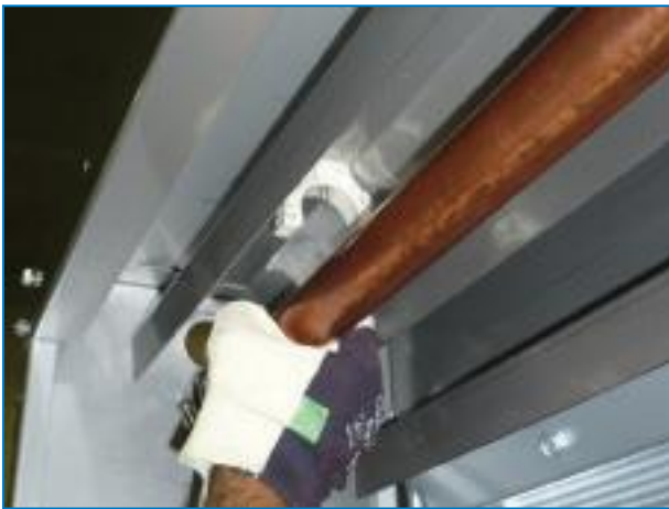
Release Copper Collector from Plastic Holders
