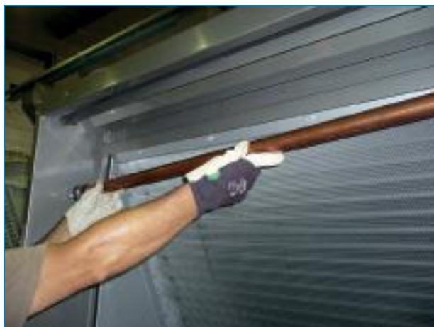
Remove Copper Waterfeed Pipe
