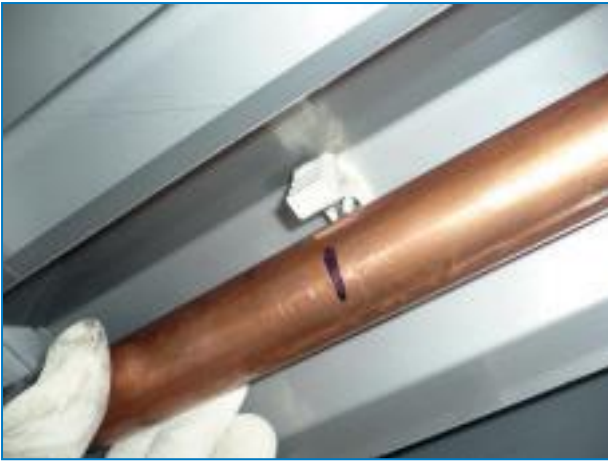
Alignment of Waterfeed Pipe
