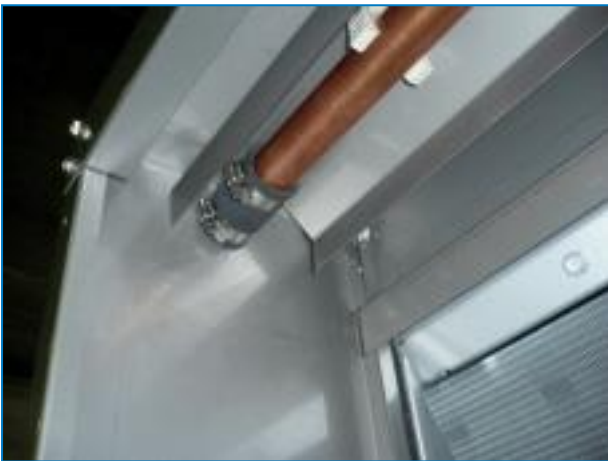
Flexible Sleeve Connection
