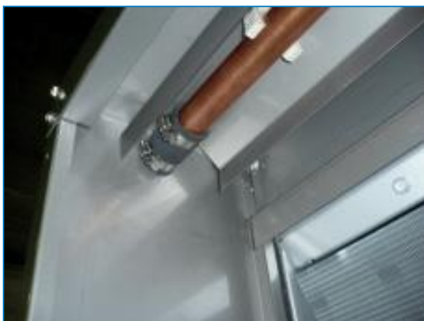
Flexible Sleeve Connection
