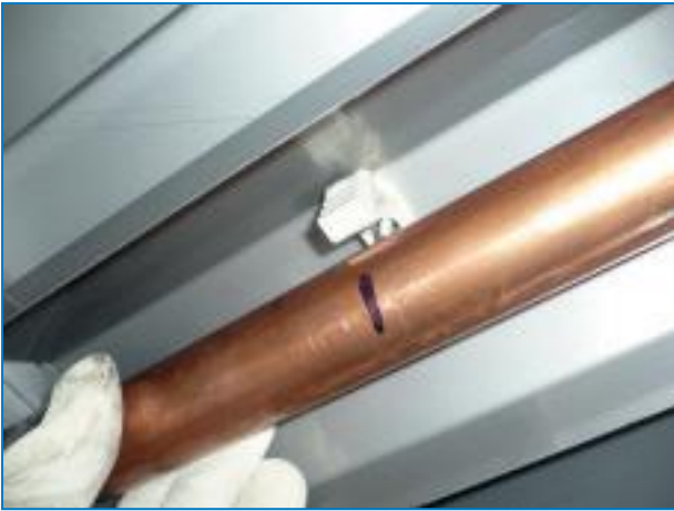
Alignment of Waterfeed Pipe
