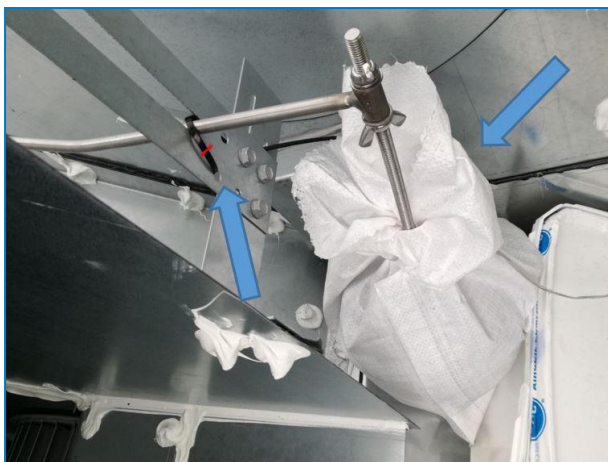
Fixation and wrapping of Float ball
