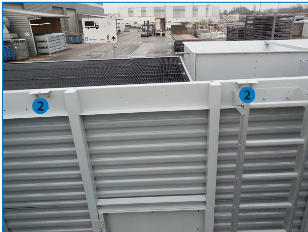
2. Rigging guide/bracket of lower section
