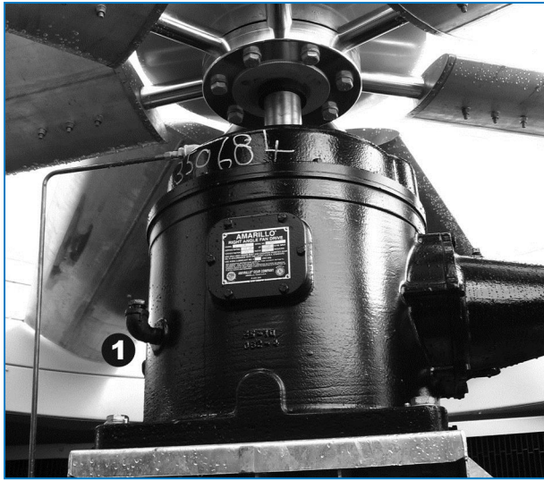
Single Reduction Gear Drive
