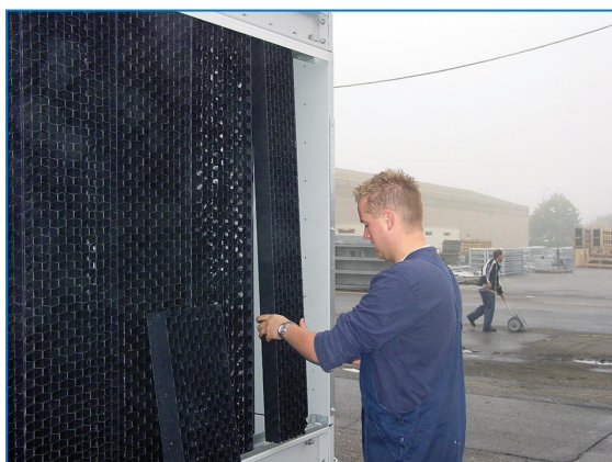
Remove Combined Inlet Shields
