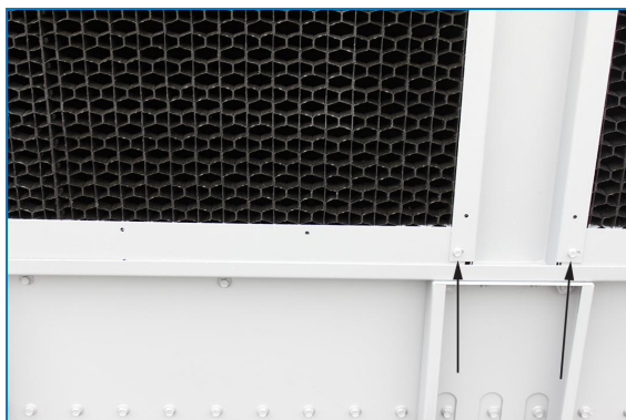
Removing Shipping Straps
