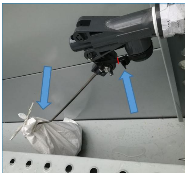
Fixation and wrapping of Float ball
