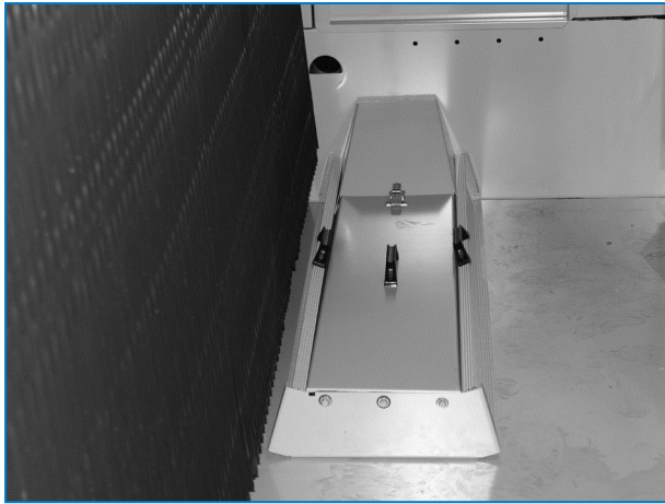
Cold Water Basin and Basin Strainer
