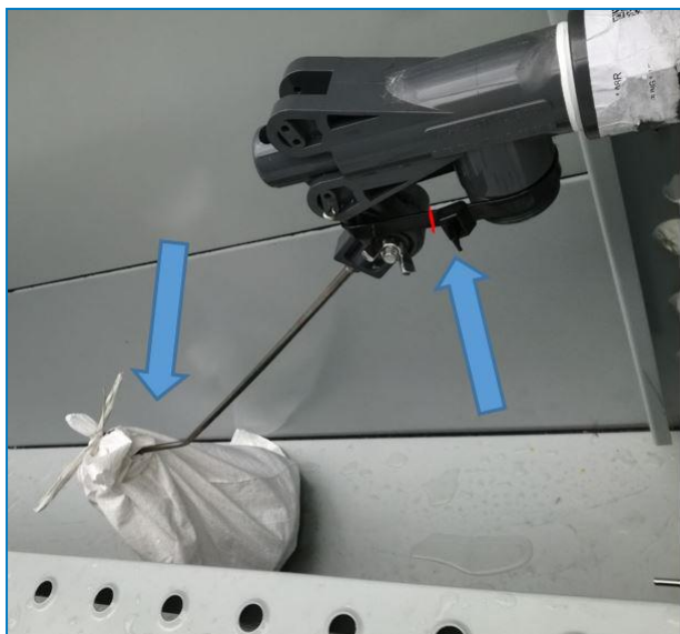
Fixation and wrapping of Float ball
