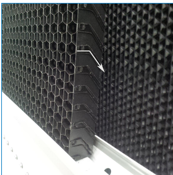
Orientation of the combined inlet shield
