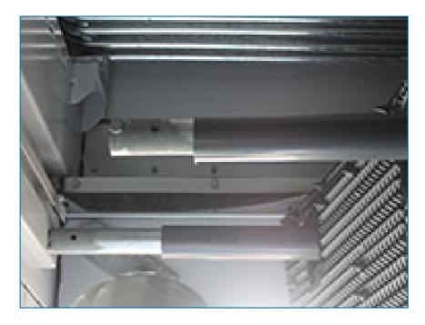
The use of telescopic fill support beams facilitates the removal and replacement of the fill sheets.
