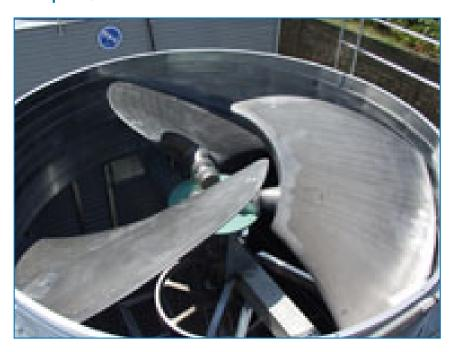
**Quiet and economical kW axial fans** mean FCT cooling towers make little sound. To reduce noise still further, choose the **Whisper quiet fan** alternative targeting optimal noise-reduction, with an aluminum hinged-blade design and unique end caps.
