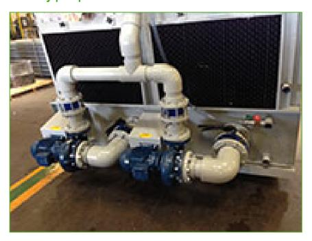
Installing a standby pump **guarantees year-round reliable operation** – the redundant pump takes over in event of a failure.
