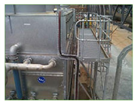
**Platforms, a ladder, safety cage and handrails** facilitate **easier and safer access** to the top level of the unit, making inspection and maintenance easier and conforming to safety standards.
