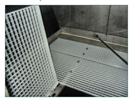
As well as **easy access to internal unit tops**, the installed internal platform also means easier and **safer** inspection and maintenance, in line with **European and South African safety directives**.
