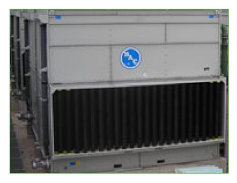
HXI hybrid closed circuit cooling towers use **quiet and low kW axial fans**, but to reduce noise even further, you can extend your HXI cooling tower with <u>sound attenuation</u>: cylindrical baffles at the air intake.
