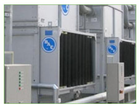
FXVE closed circuit cooling towers use **quiet and low kW axial fans**, but to reduce noise even further, you can extend your FXVE cooling tower with <u>sound attenuation</u>:
