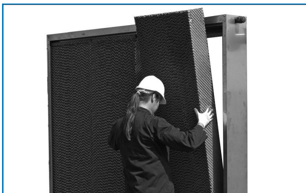
Removal of pre-cooler media
