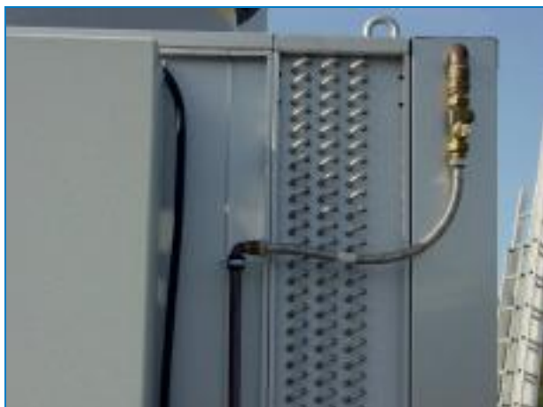
Connection of Pre-Cooler water inlet to the pre-installed copper water distribution piping.
