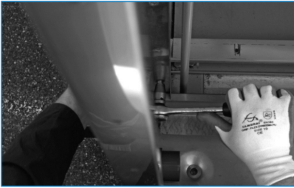
Attaching Pre-Cooler frame to dry unit with stainless steel hardware.
