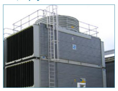
A ladder, safety cage and handrails are all installed for **easy access to the unit top and easier and safer** inspection and maintenance, in line with **European and South African safety directives**. Units equipped with these options, have also <u>distribution basin covers</u>.
