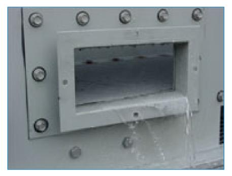
A factory-installed clean out port
